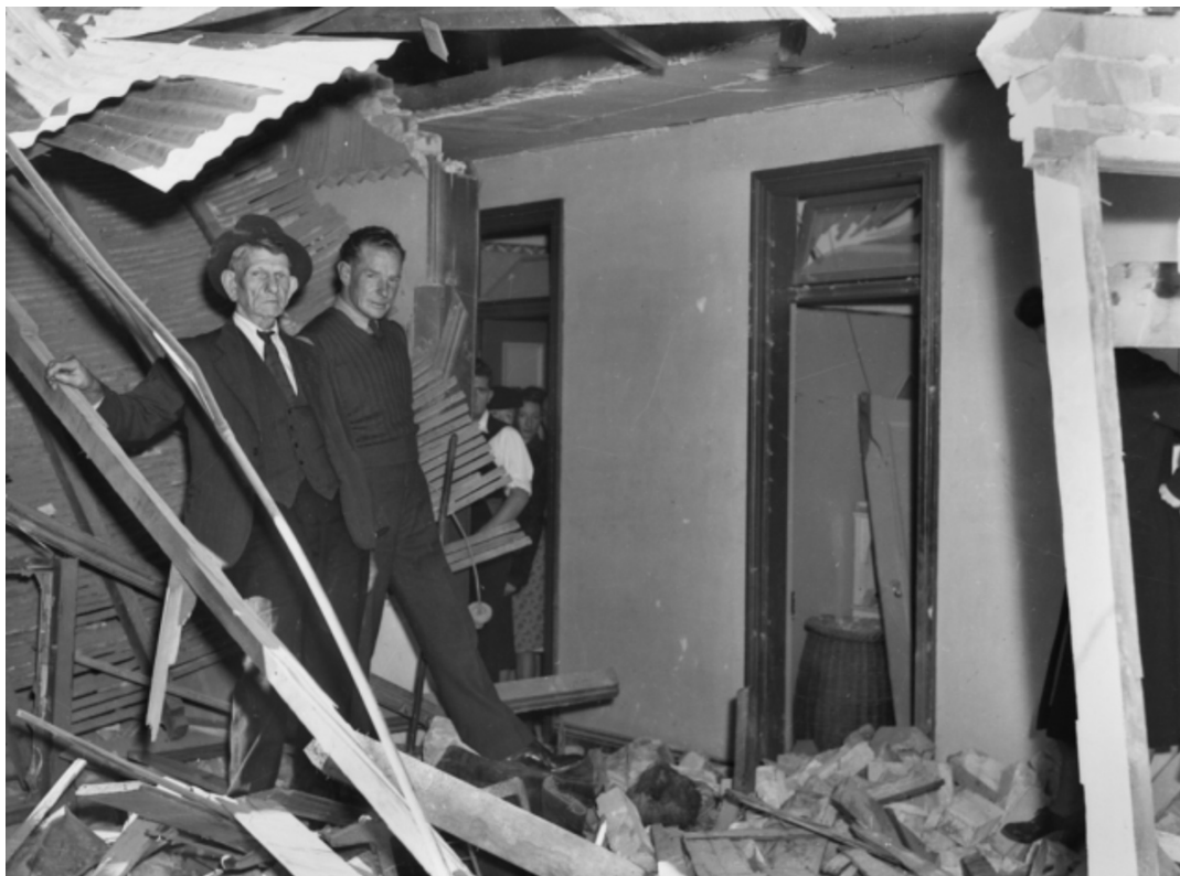
Badly damaged rear of house at 4 Bradley Avenue, Bellevue Hill.
