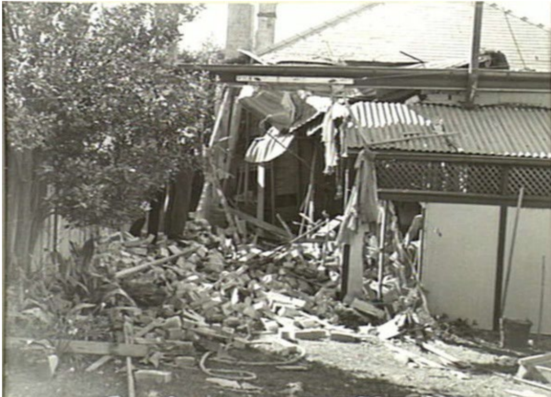
Badly damaged rear of the house at 4 Bradley Avenue, Bellevue Hill, 1942. Australian War Memorial No: 012595.
